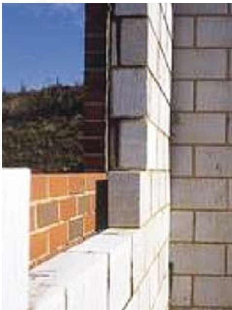
Fig1—Modern brick/block cavity wall
