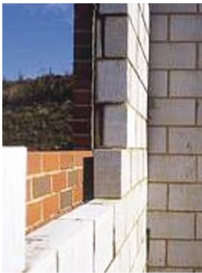
Modern cavity walls under construction.
